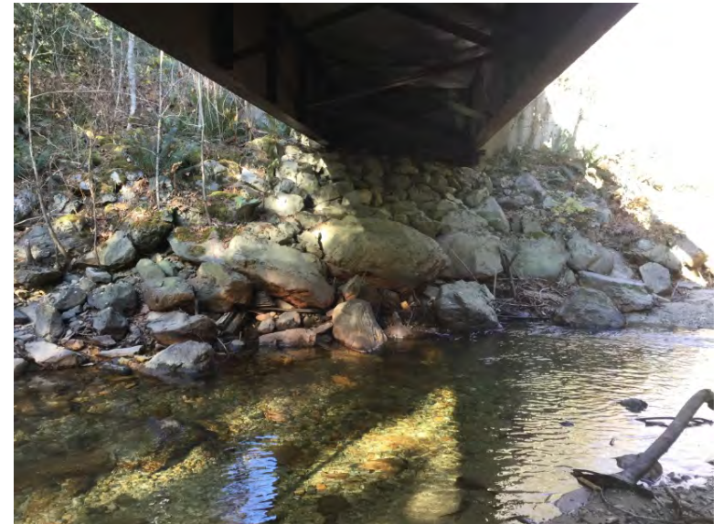
Right Bank Abutment when facing downstream
