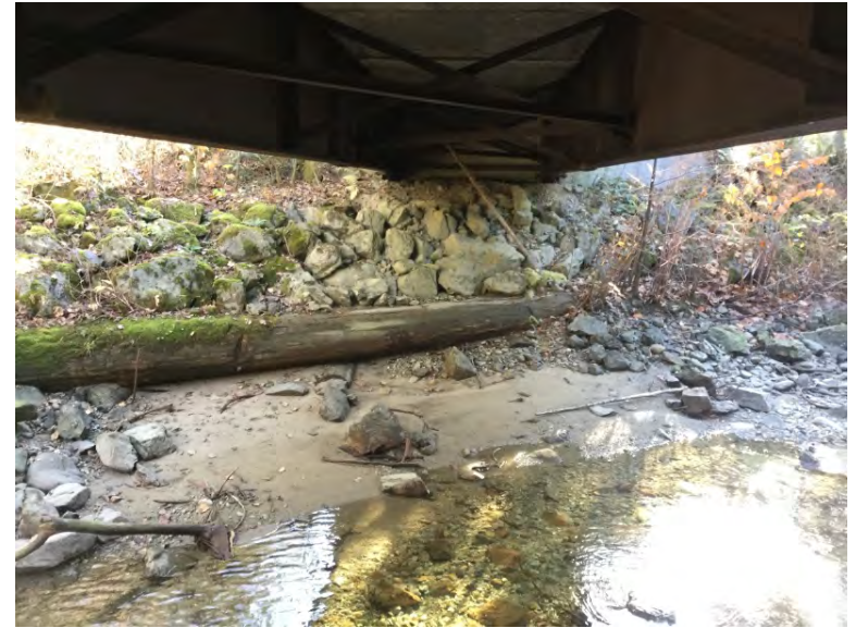
Left Bank Abutment when facing downstream
